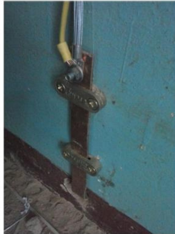
Connecting a solar system to the ground electrode
